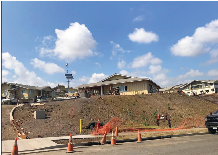
Kaiaulu development under construction.
