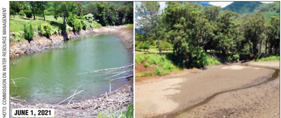
Reservoir 1, which receives water from Waikapū Stream. The southern half (right) must fill and overflow into the northern half (left) before the water level reaches a pipe that serves kuleana users.
