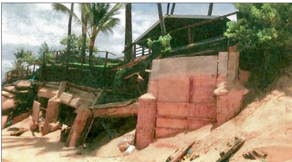
Seawall damage at the McNamaras’ Sunset Beach home following a July 2020 hurricane swell.
