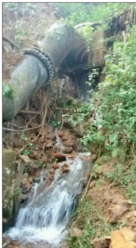
Broken siphon leaking diverted stream water in 2019.
