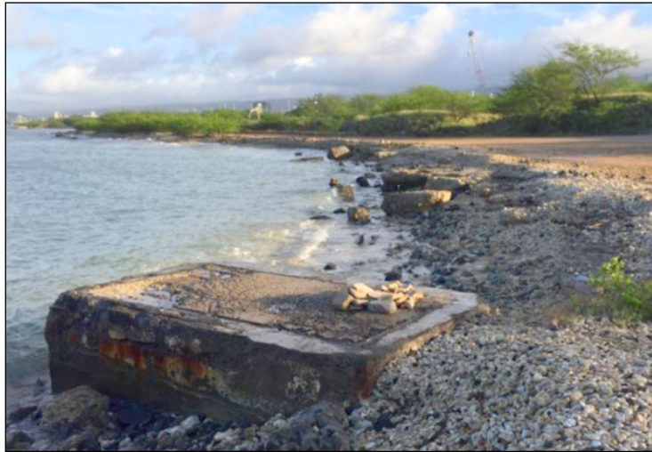
In the foreground is the stop gate for the Sand Island Wastewater Treatment Plant. Originally built 150 feet from the shoreline, it is now in danger of being inundated by waves.
