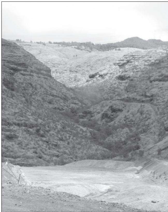
The City and County of Honolulu and Waste Management Hawai'i plan to blast out and excavate the back of Waimanalo Gulch (pictured here) to provide an estimated 15 more years of life to the city's landfill.
