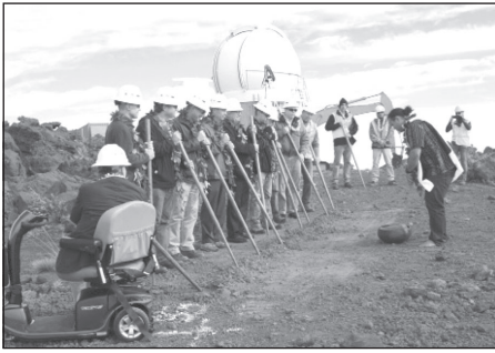
Construction of the Advanced Technology Solar Telescope on Haleakala has already begun.
