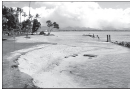
Existing shoreline near Keahi Point, looking east, showing some of the rubble placed along the shore in a failed effort to control erosion.
