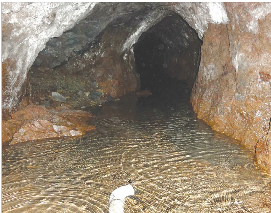
A PVC pipe collects water from one of the irrigation tunnels that serve lands in Ka‘u.
