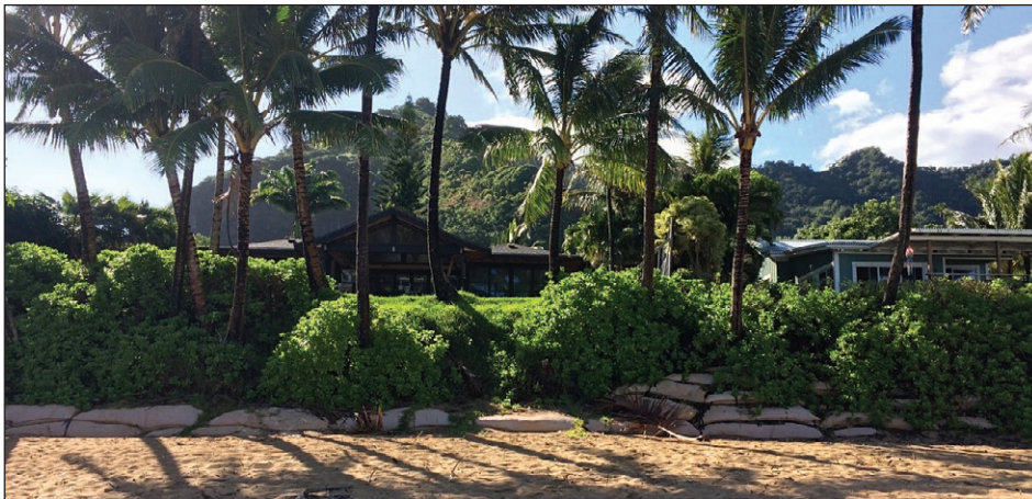
The sandbag revetment in Ha'ena, Kaua'i.
