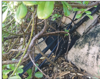
Left: A stairway with a "Private" sign at the top had been installed alongside the sandbag revetment. Above: An irrigation line hides beneath the naupaka covering the revetment.
