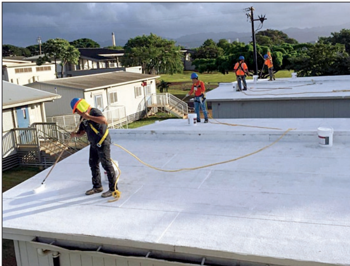
Facilities Maintenance Branch workers apply liquid coated heat reflective paint to cool more than 360 portables on O’ahu.
