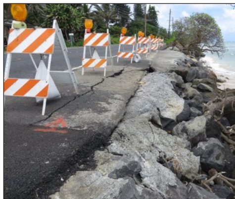
Erosion has continued to eat away at sections of Kamehameha Highway on O'ahu's northeastern coast. The two photos here were taken this summer. Left in May, right in July.
