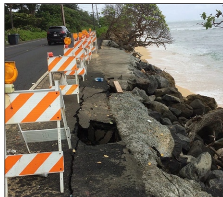
Erosion has continued to eat away at sections of Kamehameha Highway on O'ahu's northeastern coast. The two photos here were taken this summer. Left in May, right in July.
