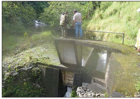
Isaac Hall argues that the East Maui Irrigation system's sluice gates, like the ones pictured here, must be enlarged to allow greater stream restoration.
