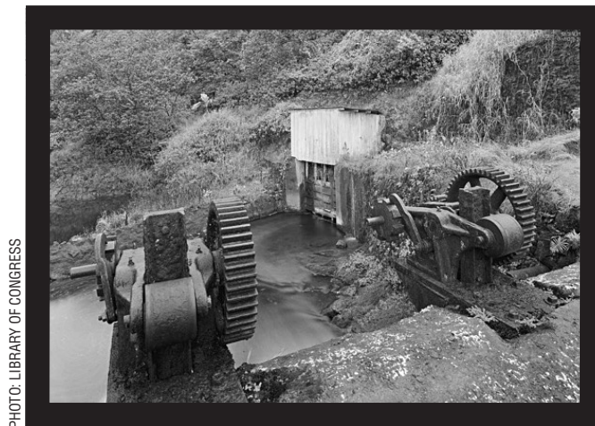
Control gates to East Maui Irrigation system in vicinity of Kopili'ulu Bridge
