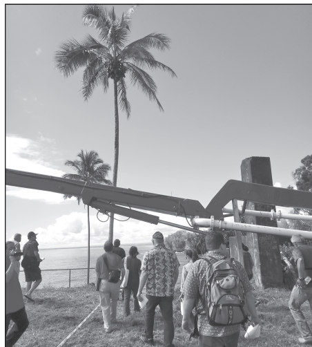
Members of the Hawai'i County Windward Planning Commission, staff, attorneys, and others visited the construction site of the "Pepe'ekeo Palace" last month.
