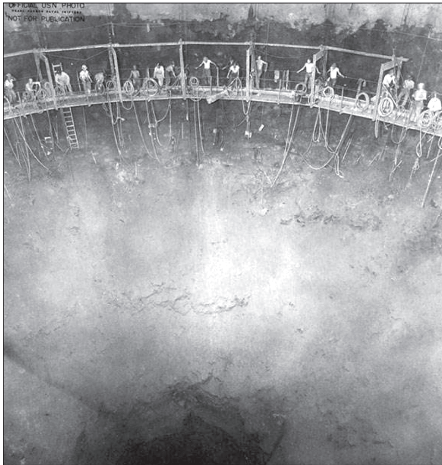
One of Red Hill’s underground storage tanks under construction in 1942.
