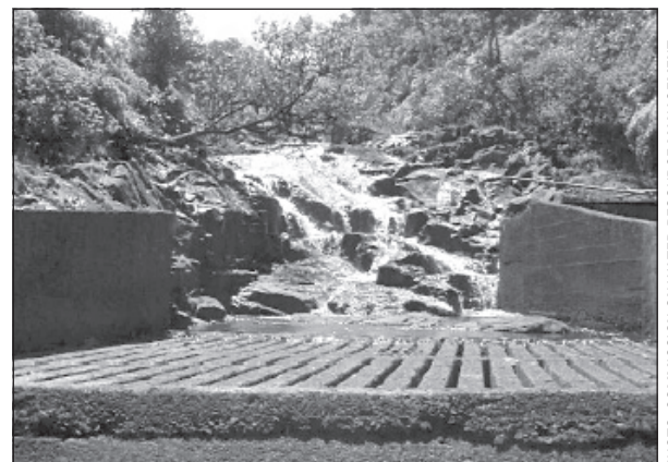
Many of the East Maui Irrigation system's diversions, like this one, are designed to take the base flow of streams.
