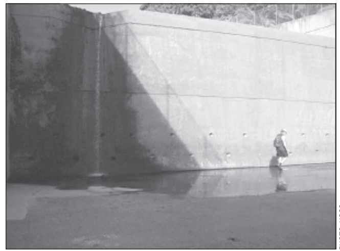
Photograph of vertical drop structure in concrete-lined channel, 'Iao Stream, Maui, Hawai'i, August 13, 2008.
