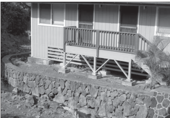
The newly built revetment alongside a stream fronting Malama Solomon's Hilo house.
