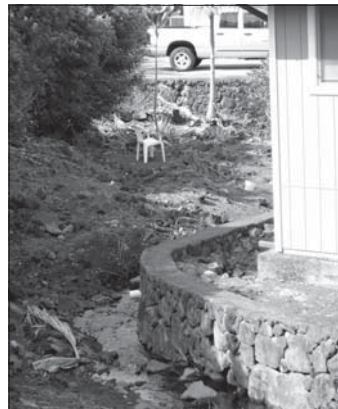
The revetment channels the stream around one corner of Solomon's house.
