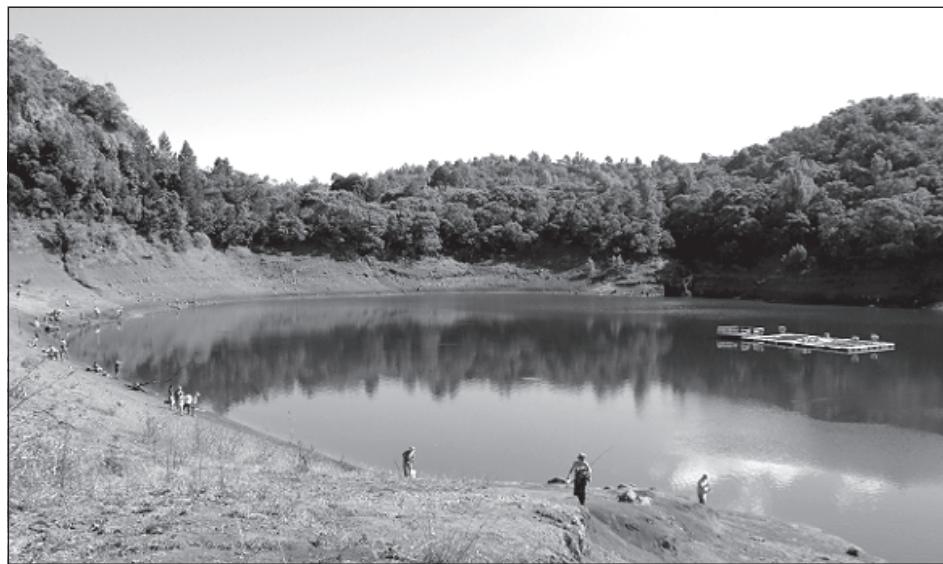
The Kaua'i Island Utility Cooperative wants to lease Pu'u Lua reservoir (pictured here) as part of a 20 megawatt pumped storage hydropower project in West Kaua'i.
